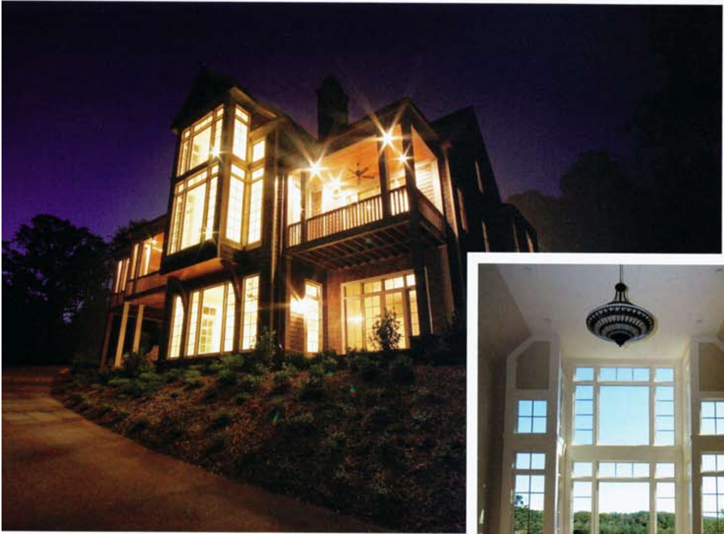
The Overlook was designed by Harrison Design Associates to take full advantage of its position on the side of a slope overlooking the river and the community.
