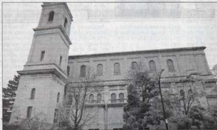
A declining neighborhood: St. Gerard's Roman Catholic Church, an 880-seat, century-old basilica that was closed two years ago, is among nearly two dozen buildings that the local diocese is trying to sell.
